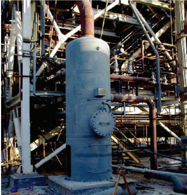
Figure 9: The Blowdown tank
