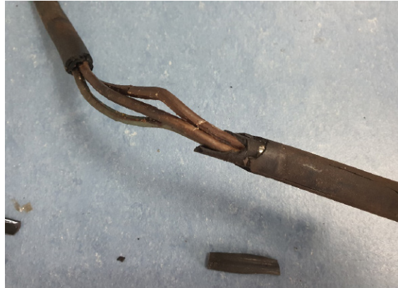
Figure 5: Part of the degraded cable sample
