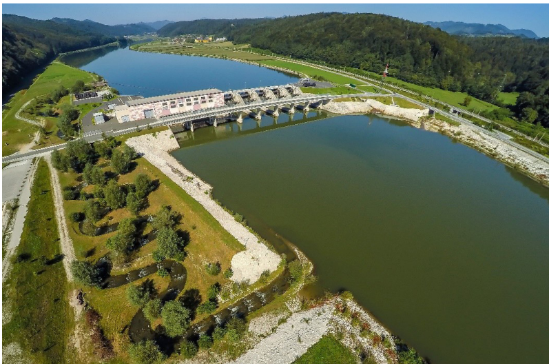
Figure 1: Fish pass next to HPP Arto-Blanca, allowing the migration of aquatic organisms.
