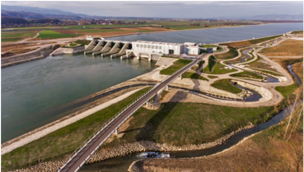
Figure 4: Brežice HPP layout with clearly visible fishway located on the left-hand-side river-bank (relative to the river flow direction) ( www.he-ss.si )
