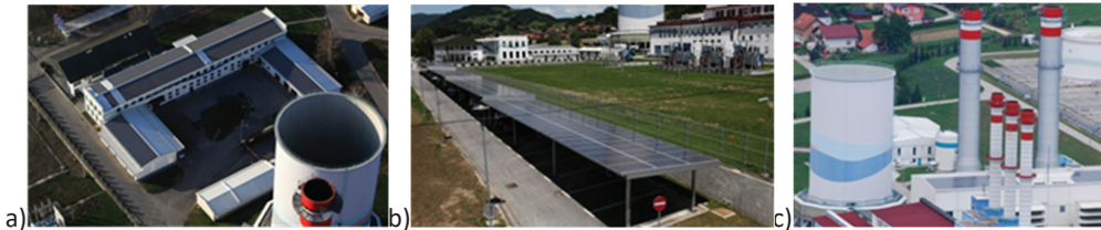
Figure 2: Photovoltaic systems MFE TEB 1-3
