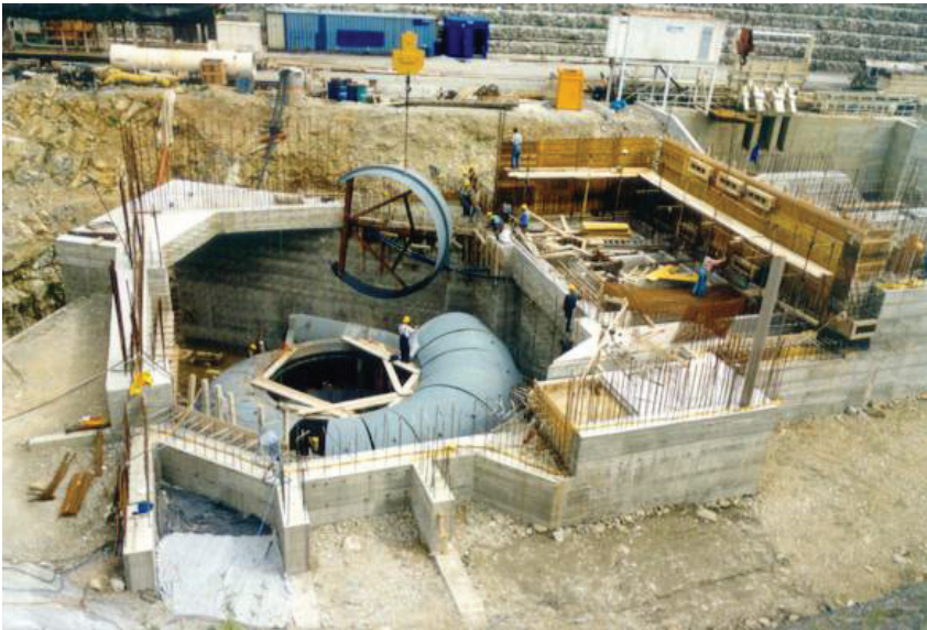
Figure 5: Plave II HPP machine hall during construction (photo Litostroj Power archive)
