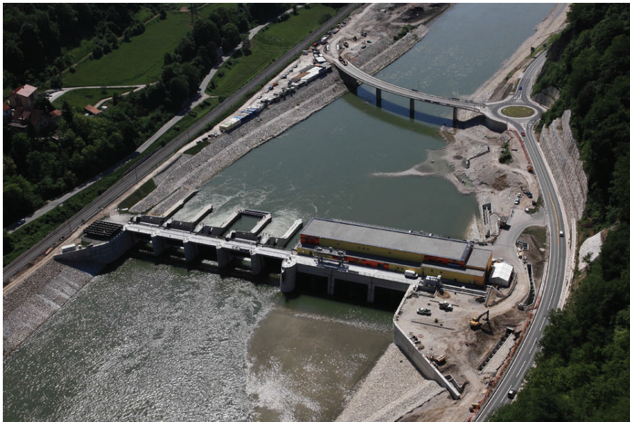
Figure 3: Krško HPP (photo Litostrój Power archive)
