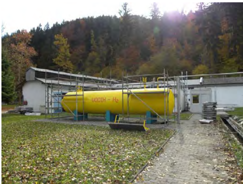
Figure 6: An example of an electrolysis plant with tanks and water pipes in the Šoštanj thermal power plant TEŠ
