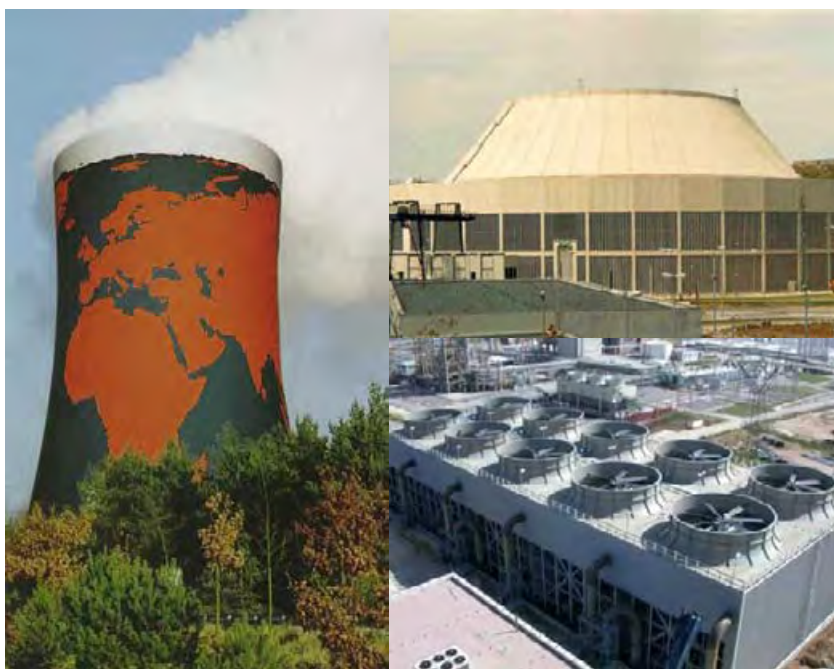
Figure 4: Cooling towers for circulating water system (CWS) and essential service water system (ESWS).
